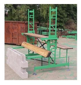
7. Deck the scaffold and store the masons' walkboards on edge as shown. This will prove to be a big timesaver. The boards will be ready when needed without having to go find them and walk them all in from the end of the scaffold. The cut-boards between towers are 80-1/2 inches long.
