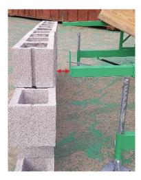
4. Space the towers about 3 fingers (2 inches) away from the footing when the masons' walkboard support (known as a "pullout" or "outrigger") is extended. The individual legs can be easily pushed or pulled into position.
