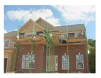
8. Add more extensions as needed following the directions in step 2. The maximum work platform height is 22'11" which is 6 extensions on the stub base tower. (WORKHORSE is actually safe over 100 feet high, but our other systems are much more practical than workhorse on walls over 16 feet high.) Our STANDARD-DUTY scaffold is shown at a job site above.
