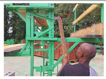
12. Remove all men and materials before lowering the scaffold. Simply push up on the holding dog and the carriage will lower to the next notch. You can lower it while standing on the ground using a 2x4 or similar object to bump the holding dog. Never climb a tower by the x-braces.
