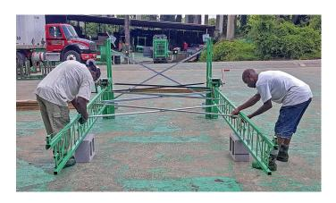
5. Install x-braces as you go. It's easier to if you stand on the outside of the towers, as shown. Be sure to start at the base and work toward the top of the tower, just like with frame scaffolding. Leave one brace out at least halfway up to give the forklift bar clearance. Check to be sure the tower will be bottom-heavy when the forklift raises it.
