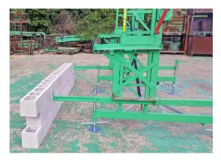
12. Space the towers about three fingers (2 inches) away from the footing when the masons' walkboard support (known as a "pullout" or "outrigger") is extended. The individual legs can be easily pushed or pulled into position.
