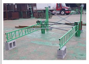
4. Move the 12" block to the end of the first extension to keep the towers from see sawing. If you wish to walk the scaffold up by hand, build the legs no higher than 17'-8" initially.
