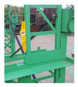
13. Plumb the tower. First plumb each individual leg, then raise the low leg of the pair by turning both leveling jacks an equal number of turns. Place your level on the tower itself to get true readings; never place it on the elevating bracket. A quality magnetic torpedo level is sufficient for plumbing.
