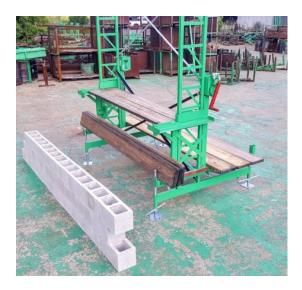
15. Deck the scaffold and store the masons' walkboards on edge as shown. This will prove to be a big timesaver. The boards will be ready when needed without having to go find them and walk them all in from the end of the scaffold. The cut-boards between towers are 80-1/2 inches long. To make the laborers' platform 4 boards, remove the snap pin on the outrigger and extend the pullout, be sure to replace the snap pin to avoid losing it.
