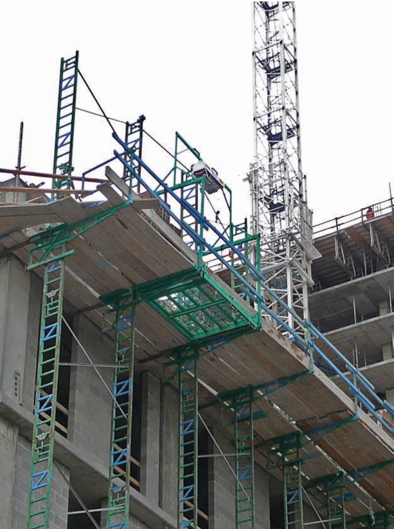
Photo 4: Materials are brought up through Non-Stop's Trap-Door with a Betamax hoist.
