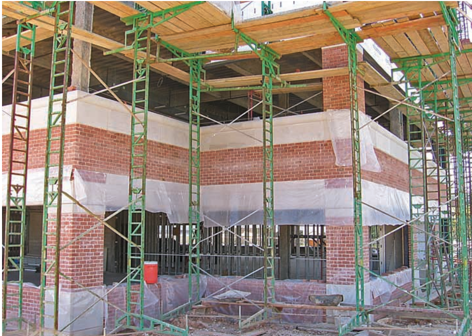
Photo 1: The tower in the corner is set first, and the others are simply set where needed to tie into the other runs.
