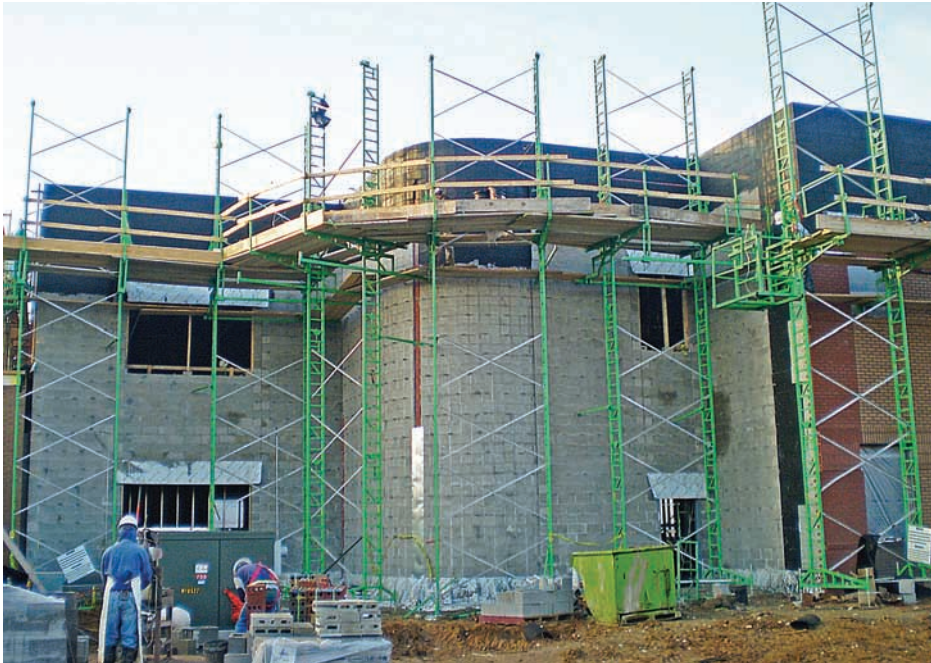
Photo 3: This complicated corner, 32 feet high, was set up in about an hour.
