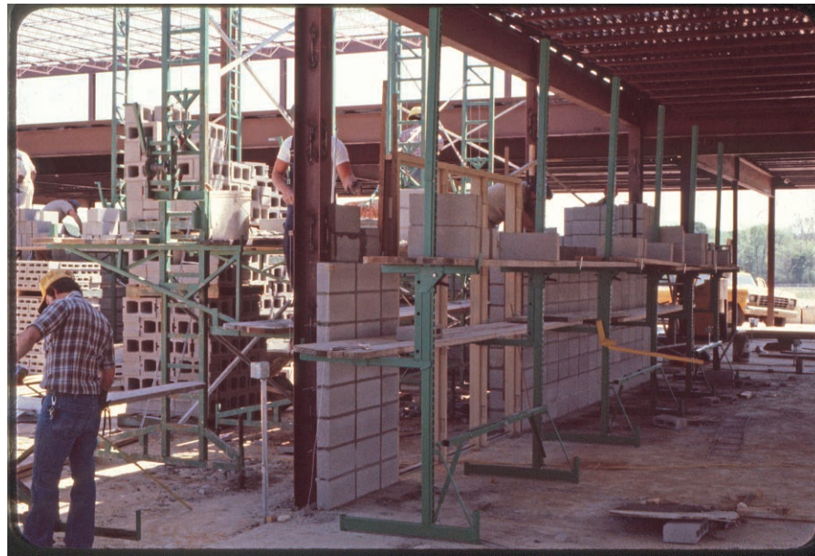
This photo was from one of Breithaupt's last jobs in 1981. The Heavy-Duty was being used inside to build a gymnasium. The very first Workhorse scaffolding is seen on the right on the corridor walls. There was nothing like it at the time, and the current Workhorse is gaining widespread popularity for interior work.
