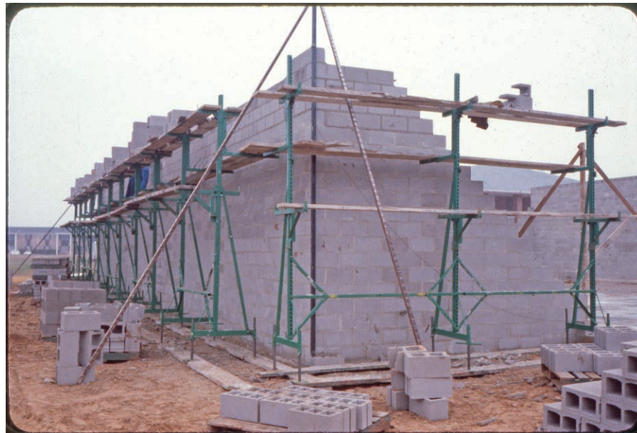
1981: Topping out an eight-inch block restaurant job on the Workhorse. Notice the speed poles set up on the corners. Ignore the lack of guardrails, etc. - this was before OSHA had made their first inspection in many areas.
