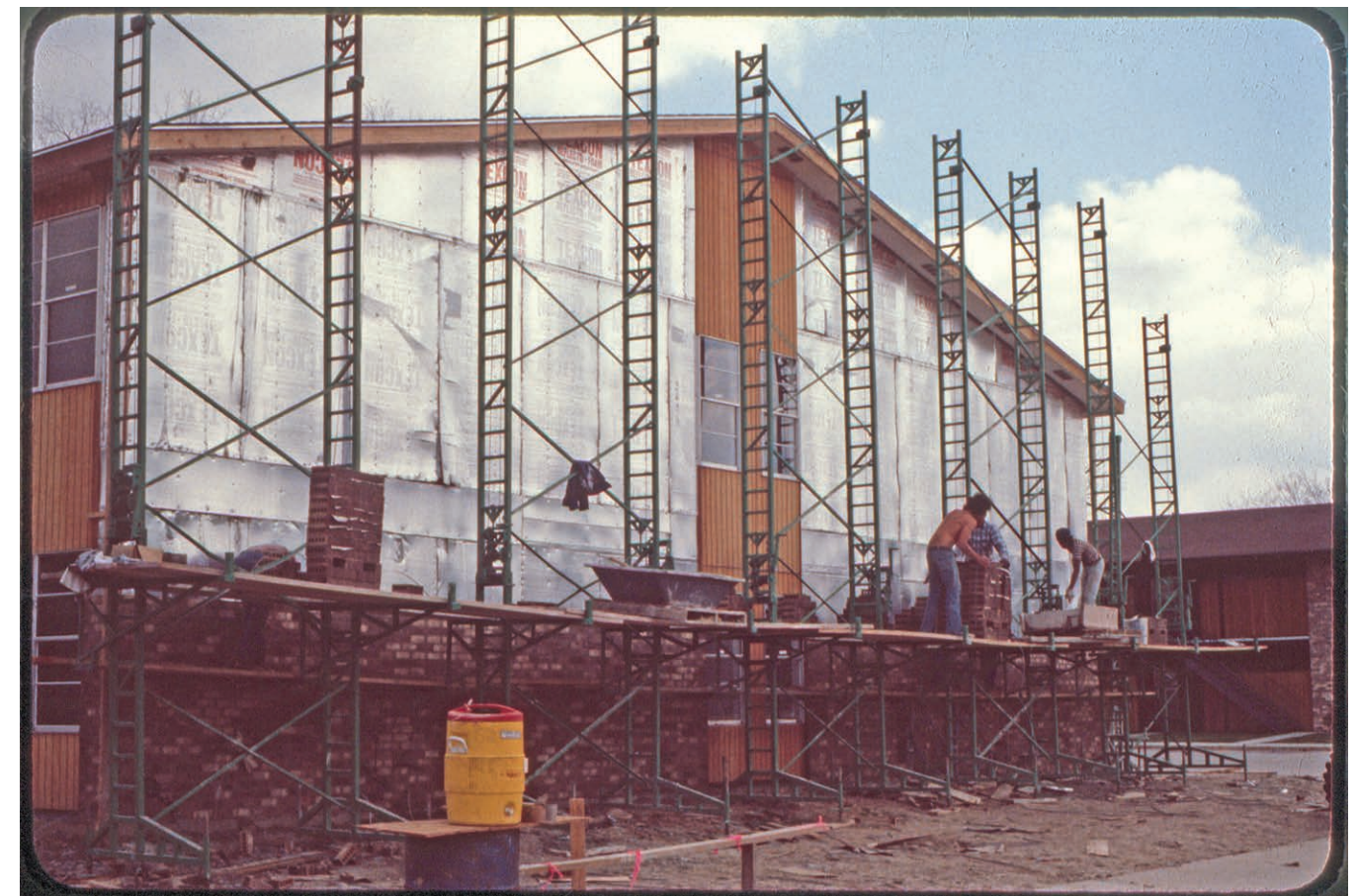
By the time this photo was taken in 1981, the Non-Stop Heavy-Duty scaffolding was gaining a foothold with contractors in seven states. Ignore the lack of guardrails, etc. – this was before OSHA had made their first inspection in many areas.
