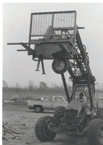
Always looking for ways to increase efficiency, Breithaupt made his own forklift wheelbarrows in the late-'70s. Notice how the wheel is shifted back under the load, instead of out front. That made it a lot easier to pick up and roll down the scaffold.
