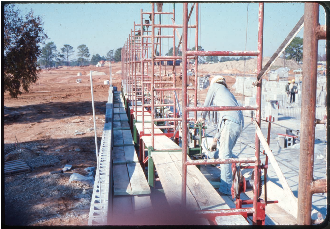
The "Old Red Scaffold" from 1971 was Breithaupt's very first elevating scaffold system. It was extremely heavy, and the lack of diagonal bracing in the towers made it a bit wiggly – two problems he designed out of future versions.
