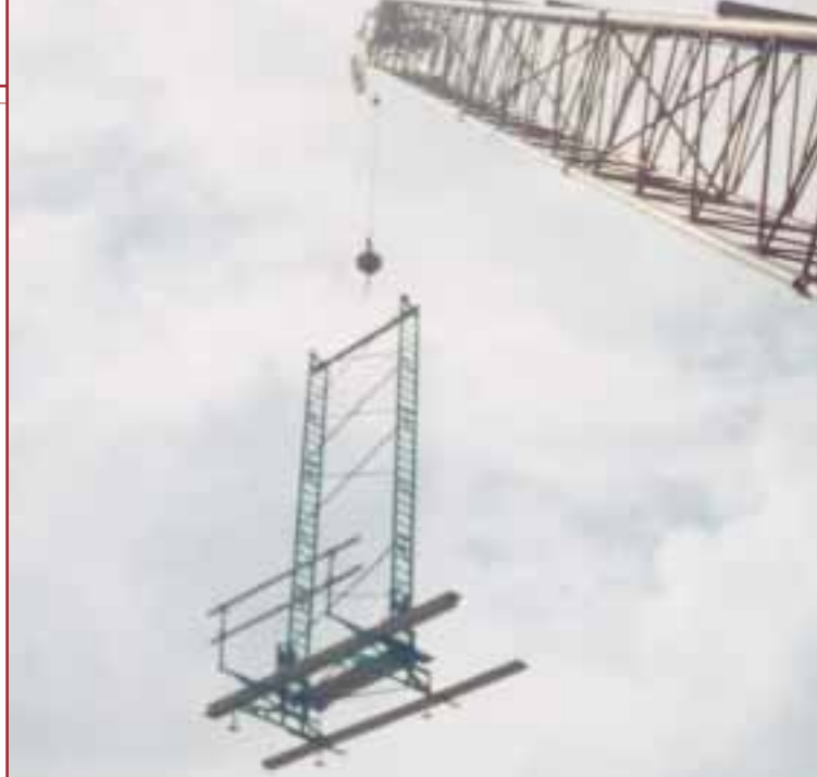
Tim Everett uses a crane to place complete towers in tough spots.
