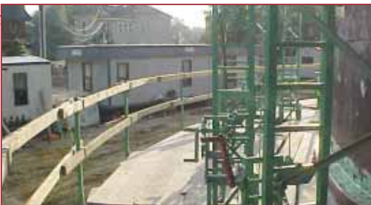
As you see here, Lucia's elevating scaffolding conforms easily to this radius wall.
