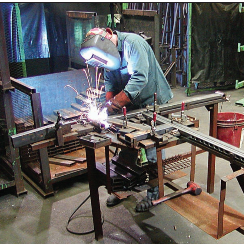
ABOVE: Welding VIP scaffold base.
