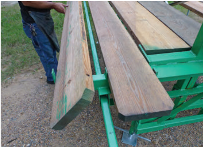
Photo 4 - An Inside Corner Arm hooks over the masons outrigger.
